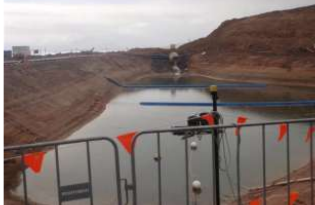
Adelaide Desalination Plant dewatering pit
