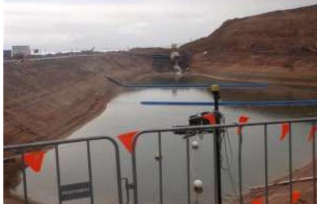
site. They had a dewatering pit – the large underground shafts were collecting 16 Litres per second, which had to be dealt with. Earthworks drainage is about control and discharge to minimise impacts as far as possible.
